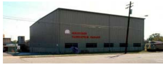
4400 Marburg Ave. Cincinnati, OH (Hamilton County)
